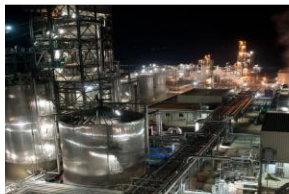
Figure 1: Beta Renewables plant in Crescentino
